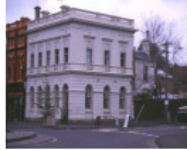
1 former bank of australasia nelson place williamstown front view jun1998
