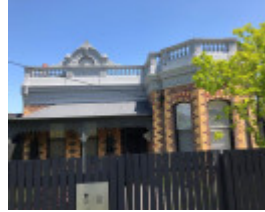
50 Stanhope Street, Malvern
