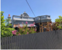
50 Stanhope Street, Malvern
