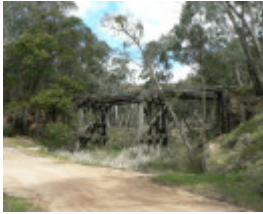
Mt Misery Creek Trestle Bridge, Berringa
