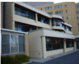
John Lindell Rehabilitation Unit 1999
