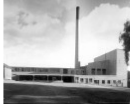
Boiler House and Laundry 1956
