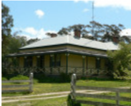
Former Mine Manager's Residence 15 Sykes Rd Berringa
