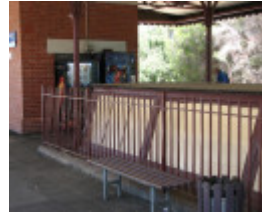
AUBURN RAILWAY STATION COMPLEX SOHE 2008
