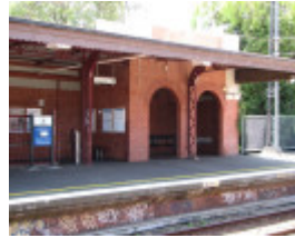
AUBURN RAILWAY STATION COMPLEX SOHE 2008
