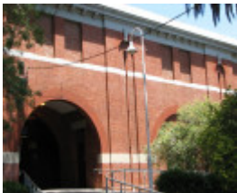
AUBURN RAILWAY STATION COMPLEX SOHE 2008
