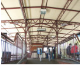
AUBURN RAILWAY STATION COMPLEX SOHE 2008
