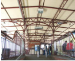
AUBURN RAILWAY STATION COMPLEX SOHE 2008
