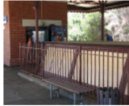
AUBURN RAILWAY STATION COMPLEX SOHE 2008
