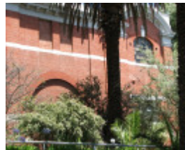
AUBURN RAILWAY STATION COMPLEX SOHE 2008
