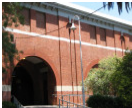
AUBURN RAILWAY STATION COMPLEX SOHE 2008
