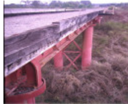
rail bridge creswick creek siding detail may1995
