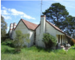
204539 11 Argyle Road, Argyle
