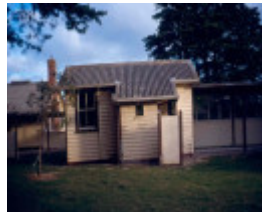
H02030 point nepean isolation hospital
