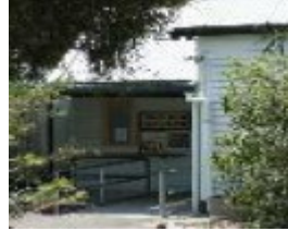
190832_Axe Creek_Patons Road_149_img02
