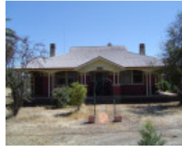
215715_Axedale_Axedale Kimbolton Road_381_img02
