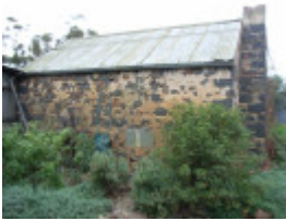
Outbuilding, 358 Brownes Lane, Axedale
