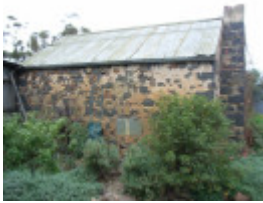
Outbuilding, 358 Brownes Lane, Axedale
