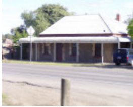
Raglan Hotel (former), 106 High Street Axedale
