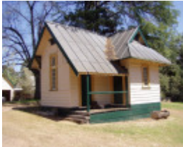
2270 Mclvor Highway, Axedale Marydale outbuildings
