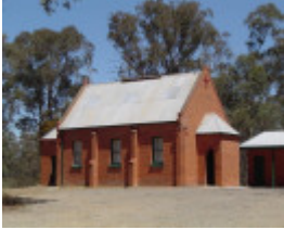
190878_Emu Creek_Hargreaves Road_108_img01
