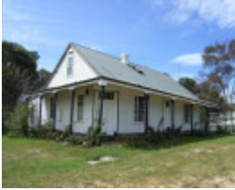
203611_Heathcote_Northern Highway South_6360_img01
