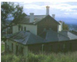
daylesford court house rear elevation jan1983
