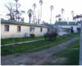
190768_Junortoun_Mclvor Highway_1044 img01
