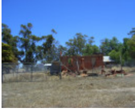
205904_Derrinal_Sheedys Lane_Murrowood Homestead_img01
