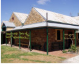
219301_Mandurang South Road_303 img 01
