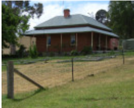
203931_Mia Mia_Valley Road_017_img01
