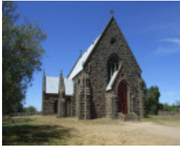
206149_Redesdale_Heathcote Redesdale Road_2115_img01
