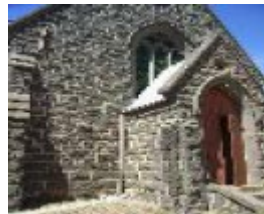
206149_Redesdale_Heathcote Redesdale Road_2115_img07
