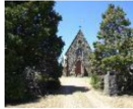
206149_Redesdale_Heathcote Redesdale Road_2115_img03
