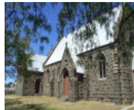
206149_Redesdale_Heathcote Redesdale Road_2115_img08
