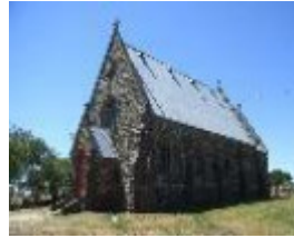
206149_Redesdale_Heathcote Redesdale Road_2115_img09
