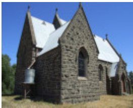
206149_Redesdale_Heathcote Redesdale Road_2115_img04
