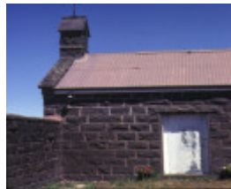
stables 1875 lara homestead derrinallum side view
