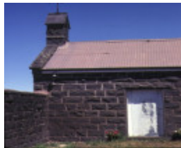
stables 1875 lara homestead derrinallum side view
