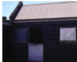
stables 1875 lara homestead derrinallum entrance
