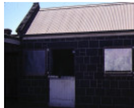
stables 1875 lara homestead derrinallum entrance
