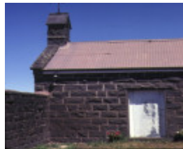
stables 1875 lara homestead derrinallum side view
