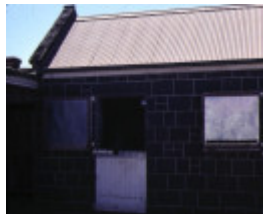
stables 1875 lara homestead derrinallum entrance
