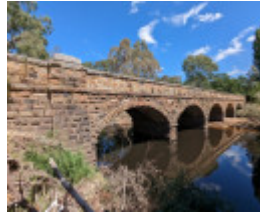
Bridge viewed from new road bridge looking south
