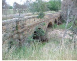
1 bridge over hughes creek avenel nov 99
