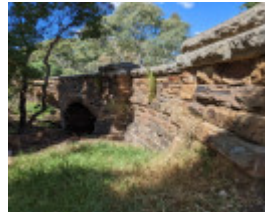
Bridge viewed from the approach looking north (?)
