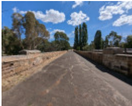
View from centre of bridge looking west
