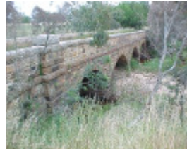
1 bridge over hughes creek avenel nov 99
