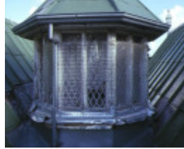
coriyule homestead mcdermott road drysdale enclosed glass room on roof
