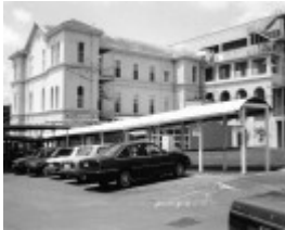
Bendigo Goldfields Hospital, Lucan Street
