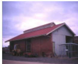
dunolly railway station goods shed may1995
