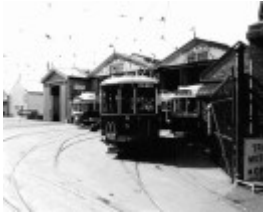
Tram Depot & Museum, Tramways Avenue
