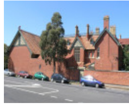
FORMER NORTH PARK SOHE 2008
