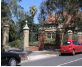
FORMER NORTH PARK SOHE 2008
