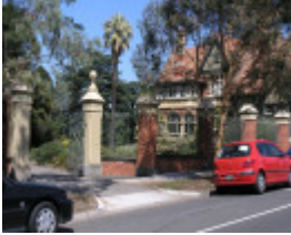
FORMER NORTH PARK SOHE 2008
