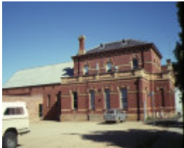
court house town hall dunolly side view
