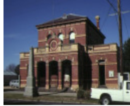
1 court house town hall dunolly front view
