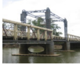
Barham Koondrook Bridge_Koondrook_Feb 2007_mz_Centre Lift Span
