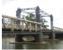
Barham Koondrook Bridge_Koondrook_Feb 2007_mz_Centre Lift Span
