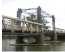
Barham Koondrook Bridge_Koondrook_Feb 2007_mz_Centre Lift Span
