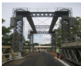
Tooleybuc Bridge_Piangil_Feb 2008_mz_Central Lift Span
