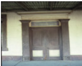
former bendigo hotel dunolly front entrance
