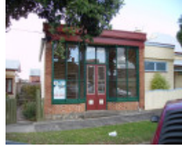
H2169 RIMG0177 - 1860 shop, 15-19 Gawler Street
