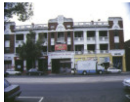
1 former number 3 carlton fire station swanston street carlton front view
