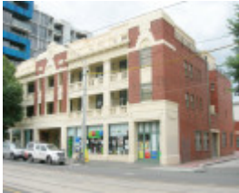
FORMER NO.3 CARLTON FIRE STATION SOHE 2008
