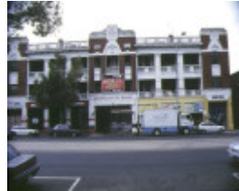
1 former number 3 carlton fire station swanston street carlton front view
