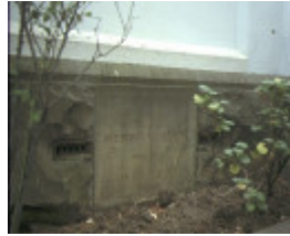
new temple church north east corner of albert street east melbourne memorial stone oct1990
