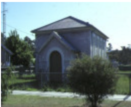
former avoca court house ballarat avoca road avoca front view nov1993
