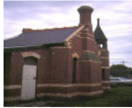
1 st albans homestead gate lodge whittington side view may1995
