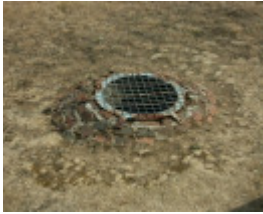
In-Ground Well, Former Hood's Bakery
