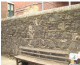
Basalt wall of coursed rubble, west boundary
