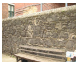
Basalt wall of coursed rubble, west boundary
