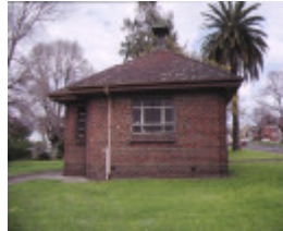
old men's shelter albert street east melbourne rear view
