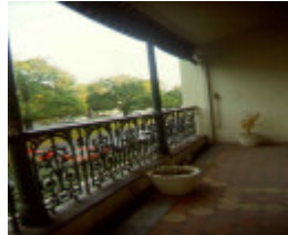
residence 206 clarendon street balcony sw apr1999
