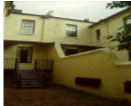
clarendon terrace rear dividing wall sw apr1999
