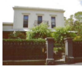
1 braemar gerorge street eat melbourne main facade jan 2000
