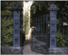
residence 193 george street east melbourne front gates may1983
