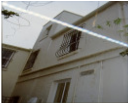
little parndon east melbourne h56 rear 1866 extension with tower room jan2000
