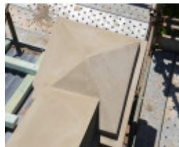
After Photograph - Reference F3878 2016
