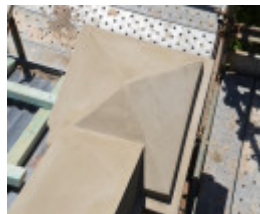
After Photograph - Reference F3878 2016
