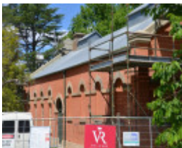
After Photograph - Reference F3878 2016
