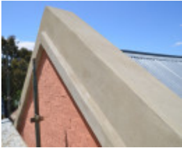
After Photograph - Reference F3878 2016
