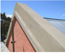
After Photograph - Reference F3878 2016
