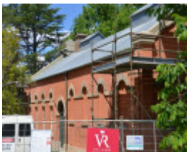
After Photograph - Reference F3878 2016
