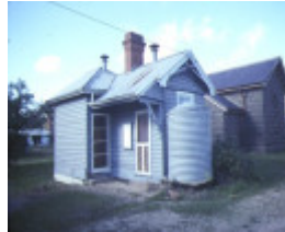
lock up davey street avoca former police station aug1984
