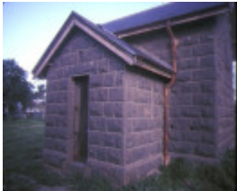
lock up davey street avoca front view aug1984
