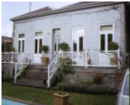
chandos 44 hotham street east melbourne rear view post1985
