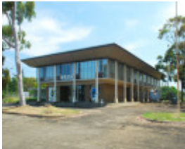
FORMER BP REFINERY ADMINISTRATION BUILDING SOHE 2008
